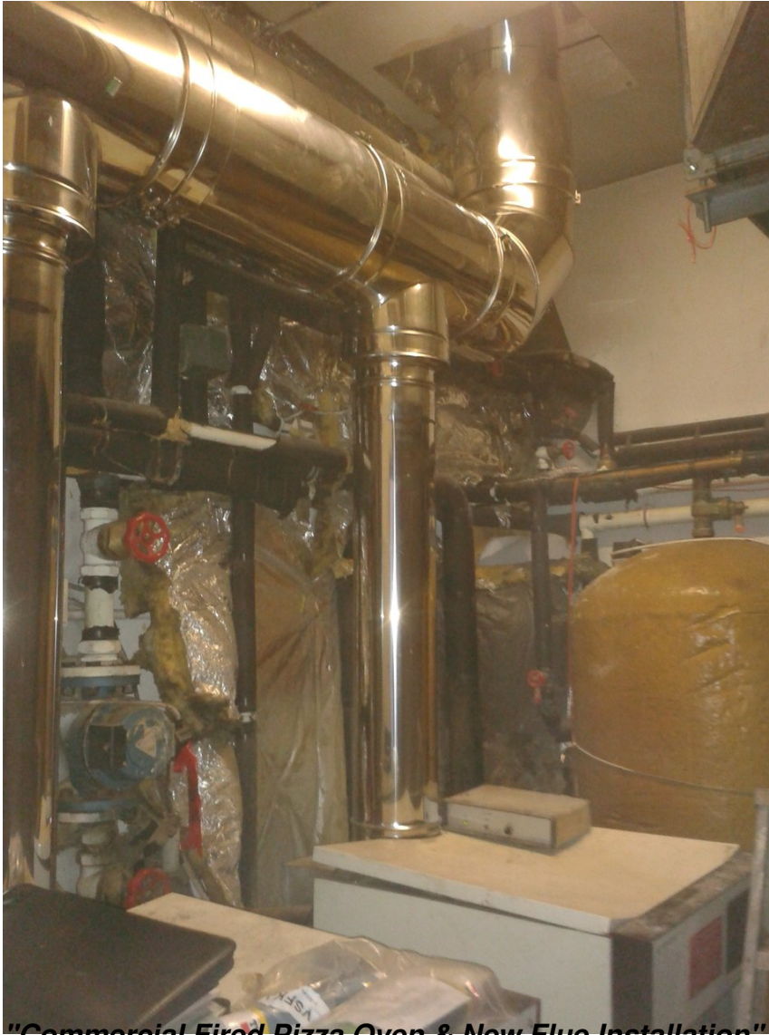
"Commercial Fired Pizza Oven & New Flue Installation"
